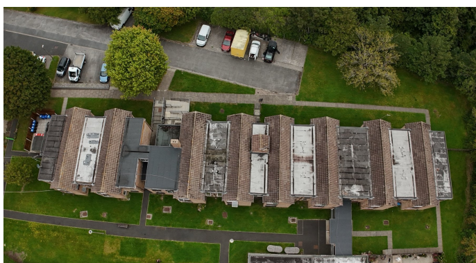
August 2025. The original flat roofs, before we started.
