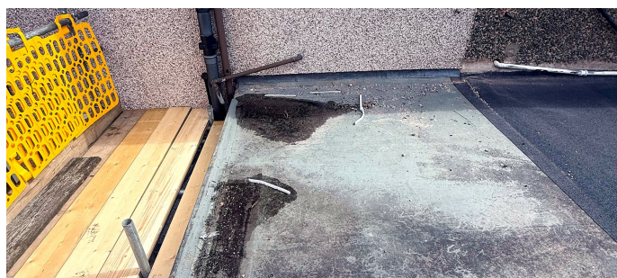
12:11. The original felt, patched and holding water.
