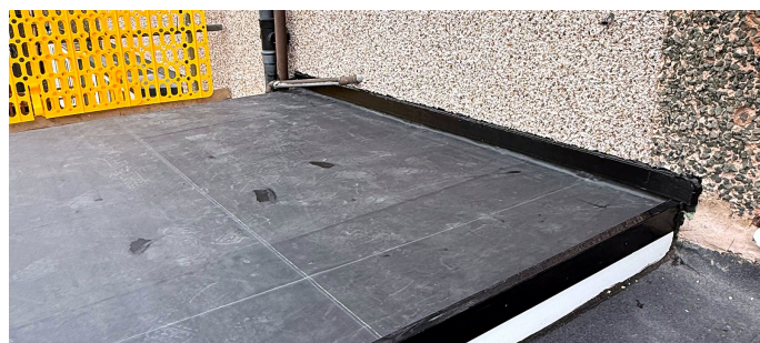
17:41. EPDM down, new edge trims on.
