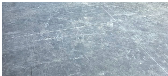
4 August. EPDM down, edges dressed, ready to hand back.
